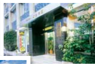
本部校舎 Headquarters building
